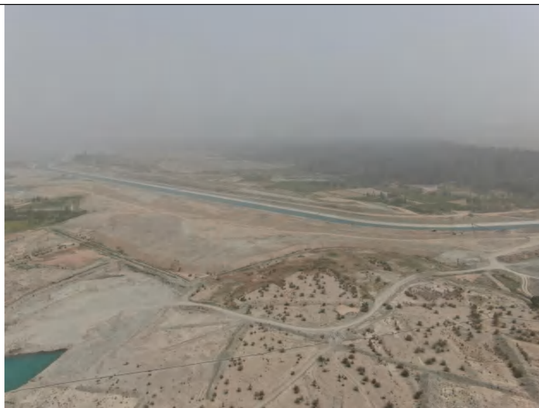
7-1#弃渣场（E76°39'29.63"，N37°53'40.91"）-南侧
