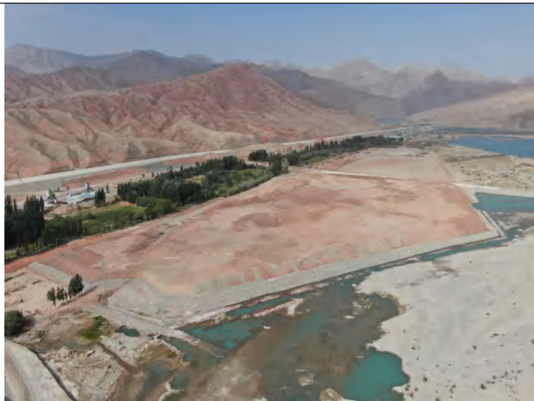
2#弃渣场 (E76°34'54.78", N 37°55'23.01") -东北侧
