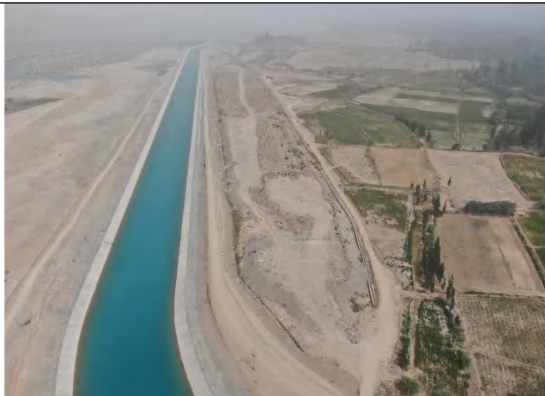
7-2#弃渣场 (E76°39'27.08", N37°53'37.68") -东侧
