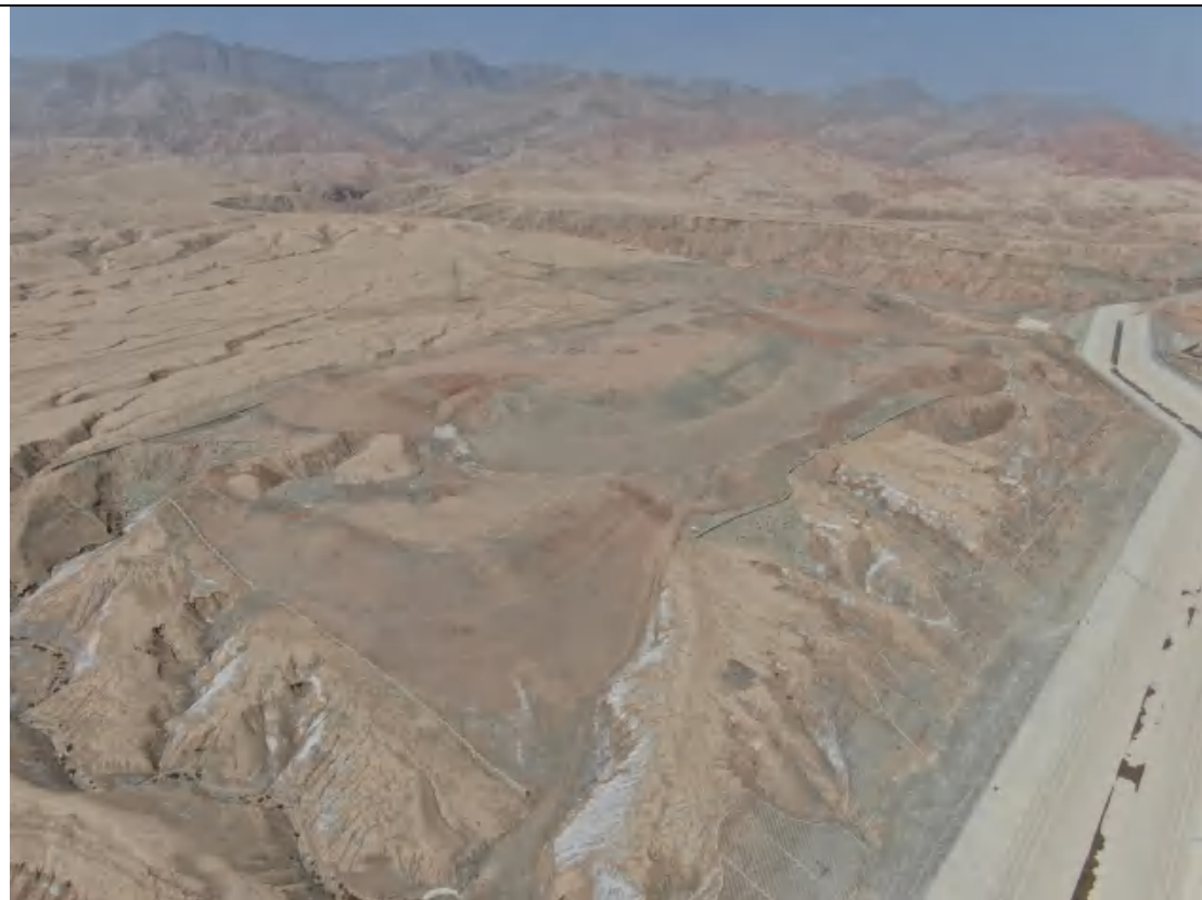
4#弃渣场 (E76°36'51.39", N37°54'8.97") -东北侧
