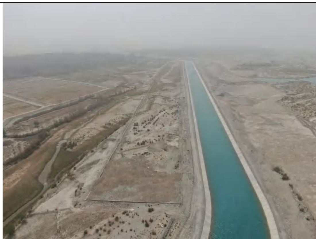
7-2#弃渣场 (E76°39'27.08", N37°53'37.68") -西侧
