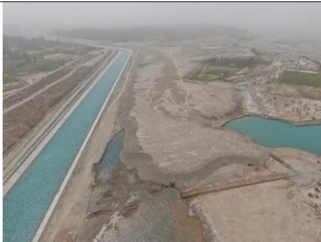
7-1#弃渣场（E76°39'29.63"，N37°53'40.91"）-西侧
