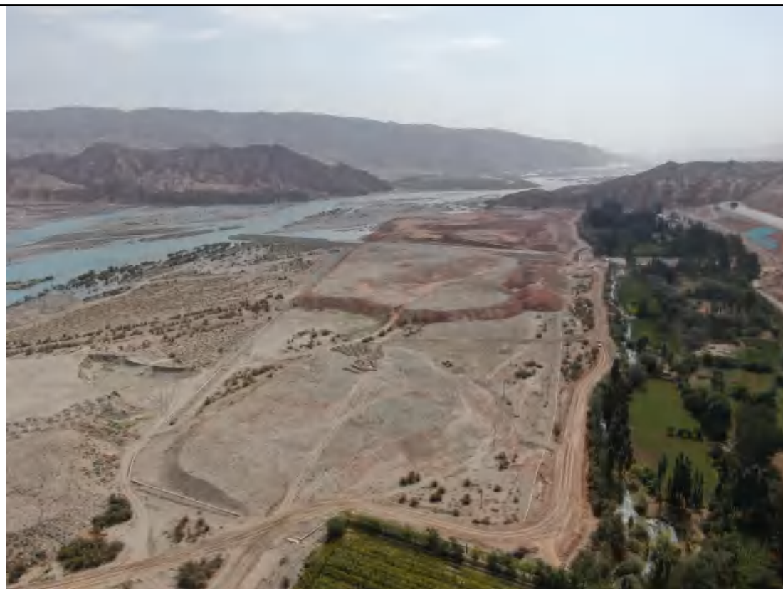
2#弃渣场 (E76°34'54.78", N 37°55'23.01") -西南侧
